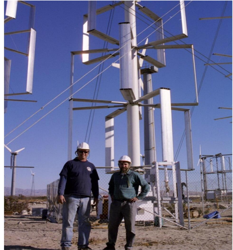
Kevin Wolf assisting with turbine installation
